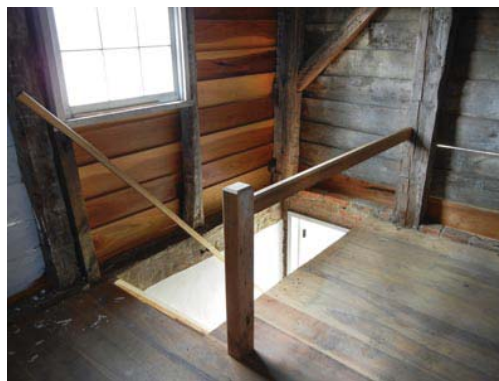
New stair rail, installed into the original mortise.
