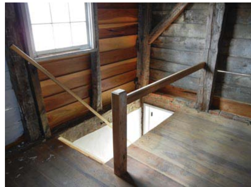
New stair rail, installed into the original mortise.
