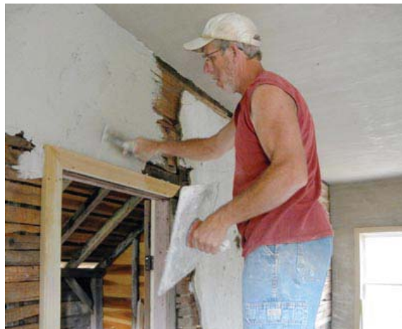
Terry putting on the scratch coat of plaster. The final surface was a thin lime coat, painted on, duplicating the original finish.
